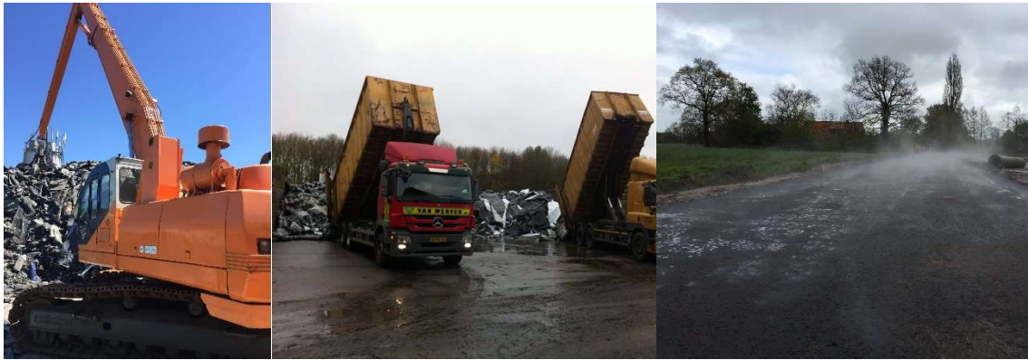
Figure 18 Recovery of roofing bitumen and recycling as road pavement
