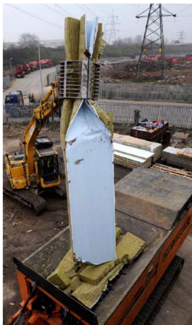
Figure 11 Recycling of mineral wool composite panels
